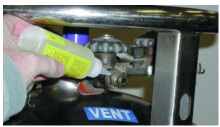
Oxygen Safe Valve Leak Check see page 8A-13 for more info
